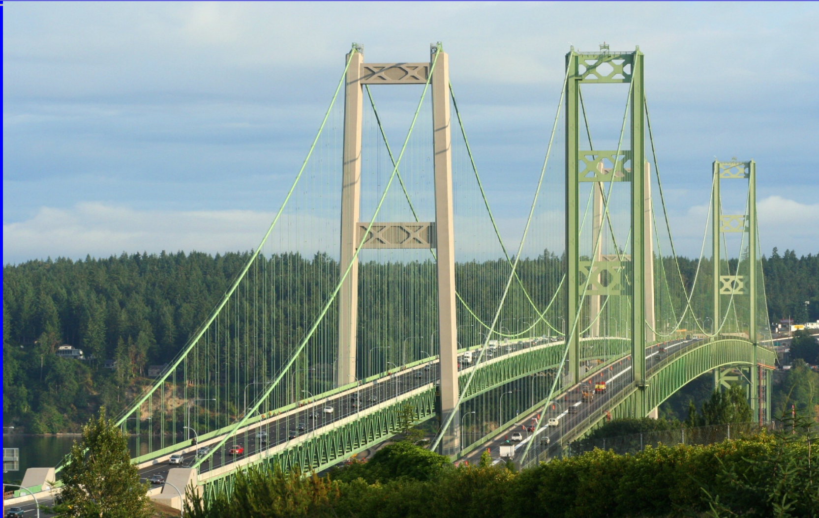
Third Tacoma Bridge, Rc pylon , truss girder, 853, completed in 2007
