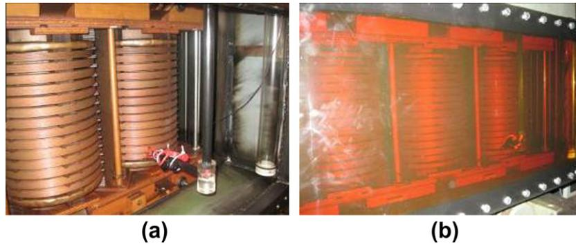
Fig. 4. Tap positions along the HV winding of the transformer, (a) before refilling the oil and (b) after refilling the oil to the tank.
